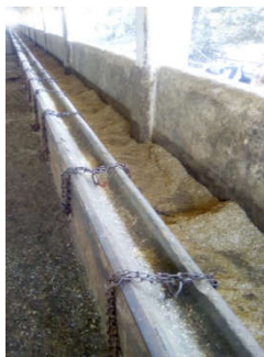
Feed bunk without partition in A Private Dairy Farm, Pariyat
