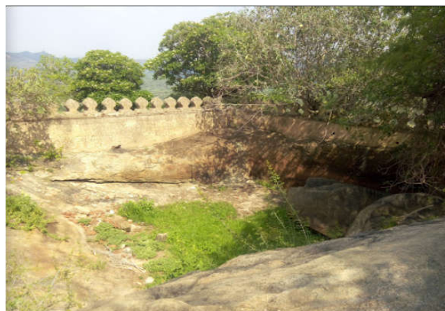
Fig 5 The Tank Edged With Brick Wall
