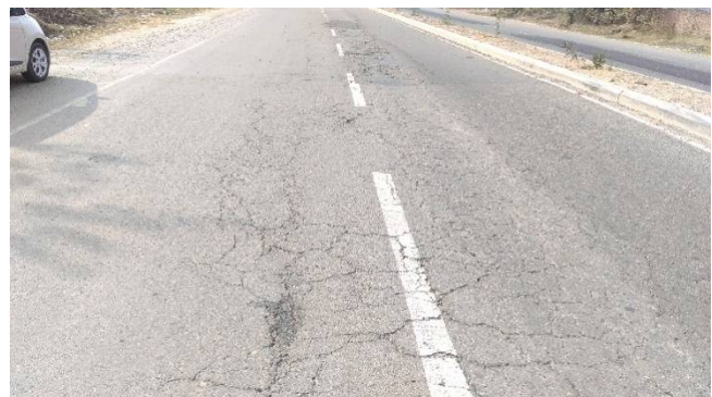
Field Condition at Chainage 14+200
