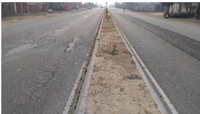
Field Condition at Chainage 11+00
