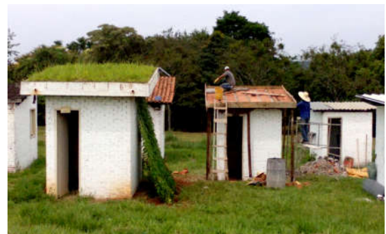
Figure 6 Construction of Green Roofs. Source: Gallardo (2017)
