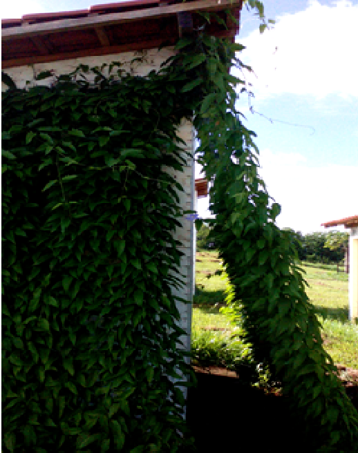
Figure 3 Plant growth on wire mesh Source: Gallardo (2017).
