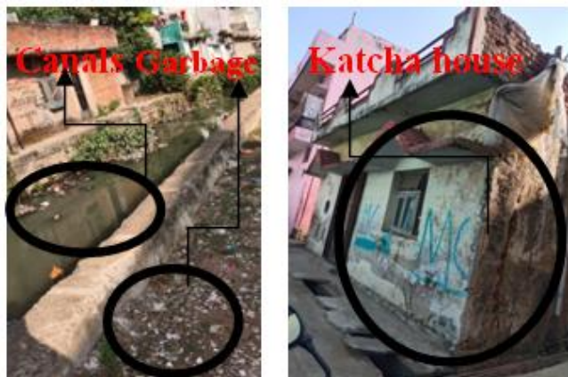
Fig 2 Existing slum in Dulari & Pujari Nagar
