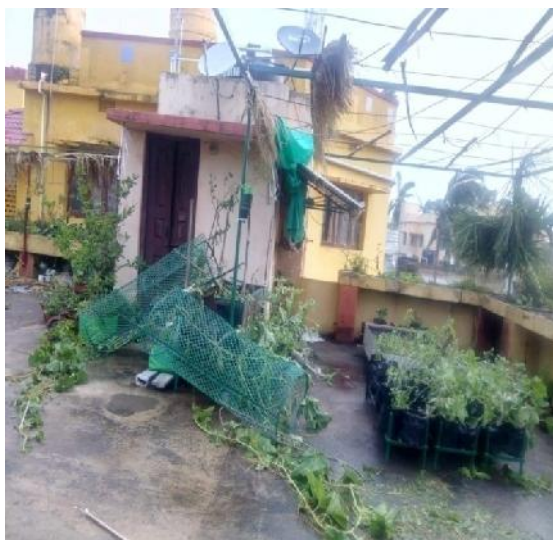
Figure 7 Severe damage of rooftop garden during cyclone fani in Bhubaneswar 2019
